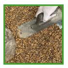
4. Compact the stones firmly to ensure a stable and flat surface. This can be done using a trowel, by applying pressure with wooden boards, or by lightly standing on the stones. This step enhances the stability suitable for foot
