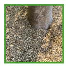
5. Leave the treated area to dry for at least 72 hours in good weather conditions. Ensure it remains dry and free from rain or frost to fully cure and harden, providing a durable and firm finish. For extra strength apply 2nd coat after 24 hours.
