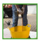
2. Thoroughly mix GravelGlue with your stones until each stone is evenly coated. This can be done using a paddle mixer, by manual shaking, or by stirring with a gauging trowel. Ensure all stones are uniformly coated.
