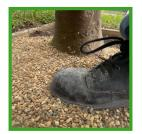
4. Allow the mixture to penetrate deeply by letting it sit undisturbed. The stones should start to bond as the mixture dries. Avoid walking on or disturbing the stones during this period.
