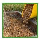
3. Pour the mixed GravelGlue and stones onto a permeable surface. This is crucial to allow drainage through the material The recommended depth for the GravelGlue and stone mixture is about 20 mm.
