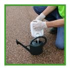
2. Pour GravelGlue into a standard watering can to ensure even distribution. Check that the mixture is well blended without any clumps to prevent clogging the spout of the can.
