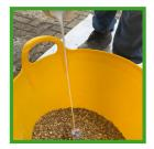
1. Combine GravelGlue with vour stones in a mixing bucket. Use one part Gravel Glue to approximately twenty-five parts stones by weight/volume (jug/bucket fills).This ratio is enough to mix 5 x 25kg bags of stones /5 litres of GravelGlue.
